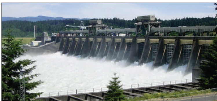
Figure 6.14: Hydroelectric power station
