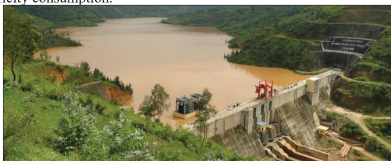
Figure 6.15: Hydro electric Power Plant Project on River Nyabarongo
